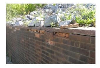
**Project Description:** The retaining wall behind the Transportation Department is deteriorating and needs to be replaced or reinforced to avoid failure in the future.
