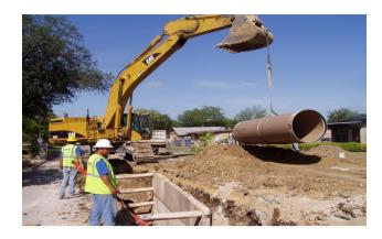
**Project Description:** Sewer system improvement in the Welcome/North Davidson area will develop the infrastructure necessary for economic growth in the area. This project includes 12" of gravity sewer, manholes, forcemain, road crossing, railroad crossing, erosion control. It also consists of ACP pump station upgrade, engineering design fees, CA & inspection, and easement acquisition.
