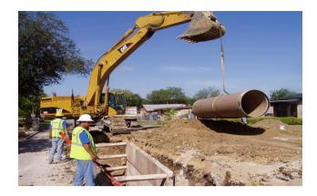
Project Description: The Southmont area business district sewer system improvements is to develop the infrastructure necessary for economic growth and development in the Southmont area. The project includes 6,400 LF of 8" gravity sewer, forcemain, manholes, air relief valve in manholes, road crossings, railroad crossings, erosion control and a pump station. Other necessary services are included in the cost of this project such as engineering fees, inspection and easement preparation.
