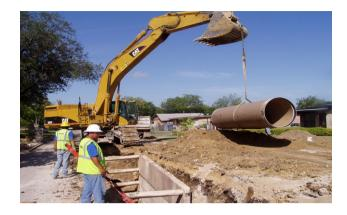
Project Description: Sanitary sewer extension and improvement on Highway 150 at Northwest Elementary School. This project includes 8" PVC Sewer and 8" DIP Sewer. It also includes manholes, service stub and clean out, stabilization stone and erosion control. Engineering fees and easement acquisition are included in the cost of this project. This project develops the infrastructure necessary for economic growth.
