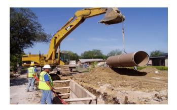
**Project Description:** Gravity sewer extension to Davis Townsend Elementary School located at 975 Heath Church Road, Lexington, NC. This project includes 8" gravity sewer, manholes, road crossings, interstate crossings, creek crossings, stabilization stone and 6,500 linear foot of erosion control. The cost estimate for this project also includes engineering and construction administration, contingencies, and legal, financial and administration costs.
