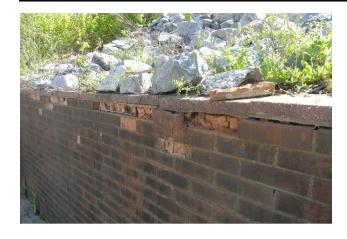
**Project Description:** The retaining wall behind the Transportation Department is deteriorating and needs to be replaced to avoid failure in the future.
