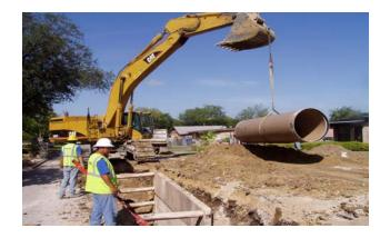
**Project Description:** The Southmont area business district sewer system improvements is to develop the infrastructure necessary for economic growth and development in the Southmont area. The project includes 6,400 LF of 8" gravity sewer, forcemain, manholes, air relief valve in manholes, road crossings, railroad crossings, erosion control and a pump station. Other
